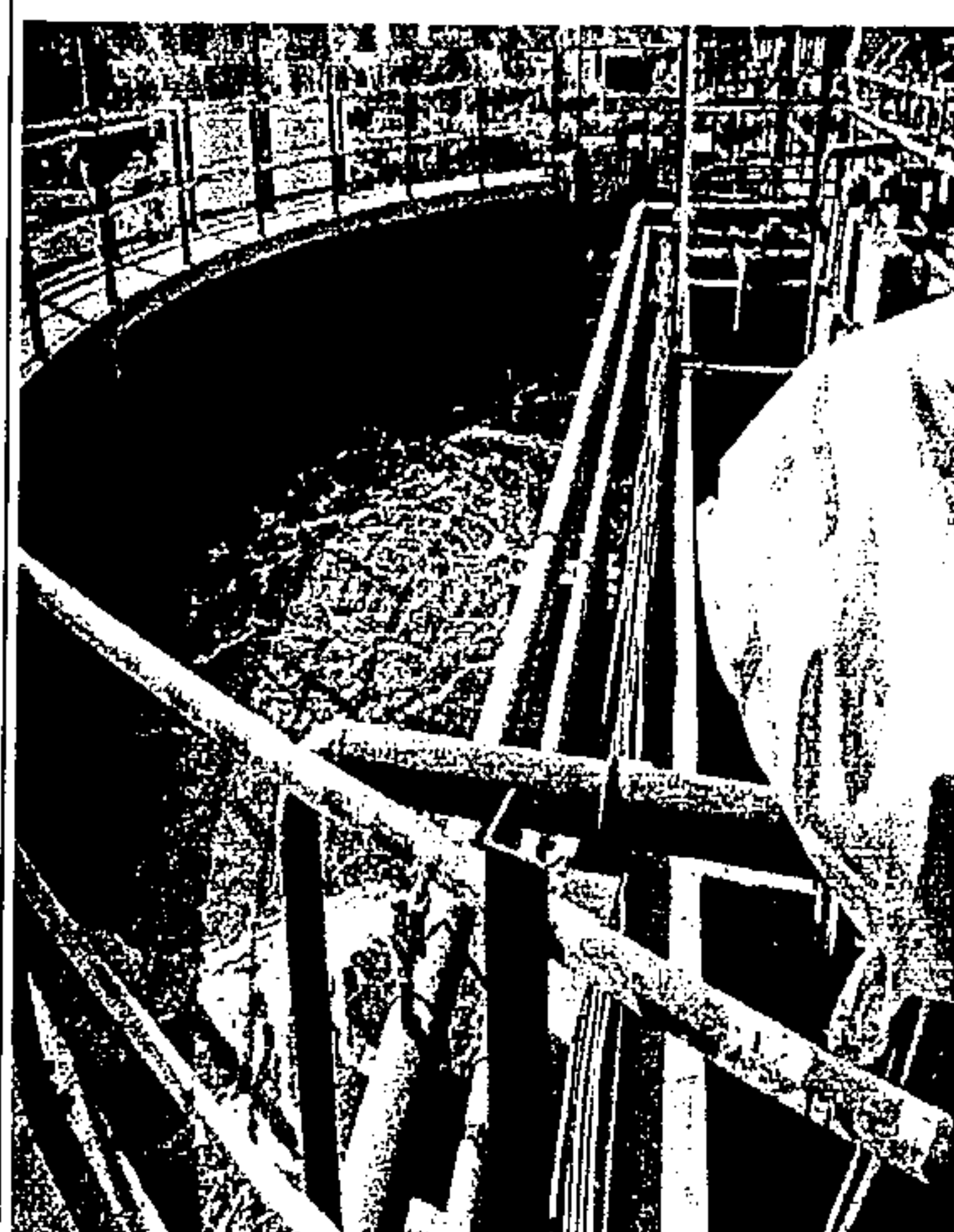
View of SBR reactor in operation
