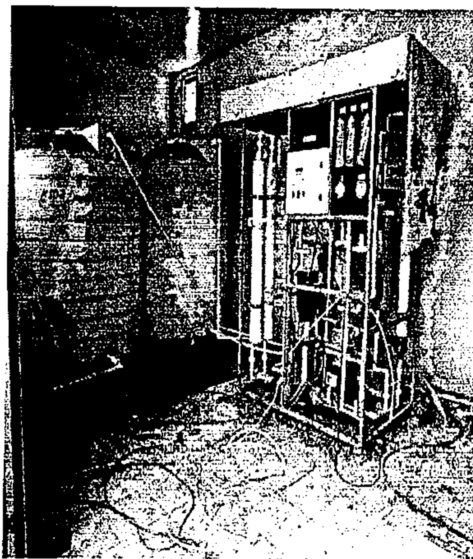
RO plant installed by PHED in the premises of Government middle school for drinking water supply to the Milakpur-Gurjar village but it was not in operation.
